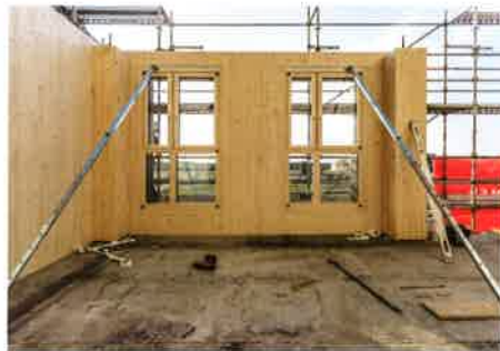
Sequence of placement and installation of the prefabricated wall panels. The bottom right image shows the installation of an interior core free-standing column.
