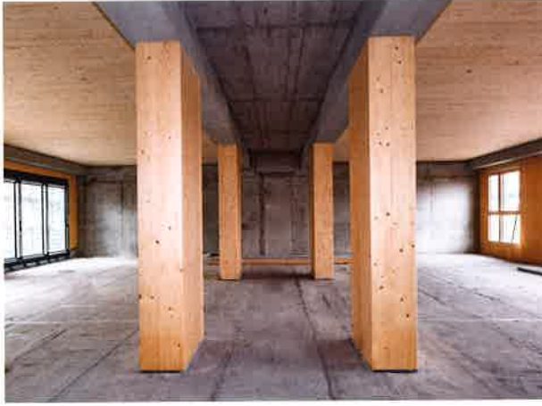
Interior precast concrete beams and free-standing timber columns, instead of concrete core walls, provide support of the floor panels.
