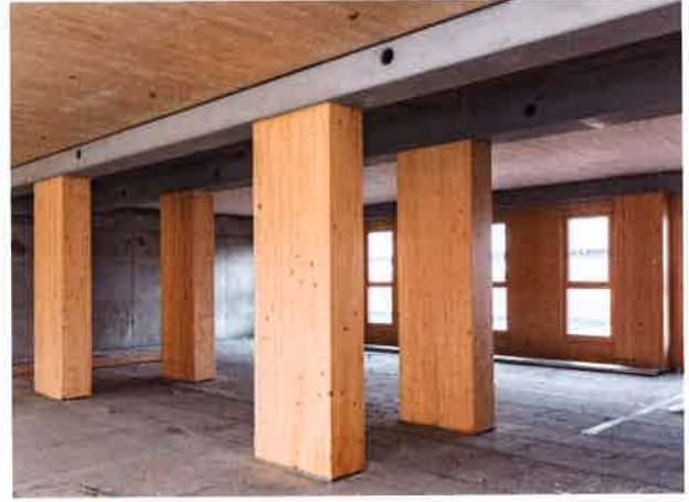
Interior precast concrete beams and free-standing timber columns, instead of concrete core walls, provide support of the floor panels.
