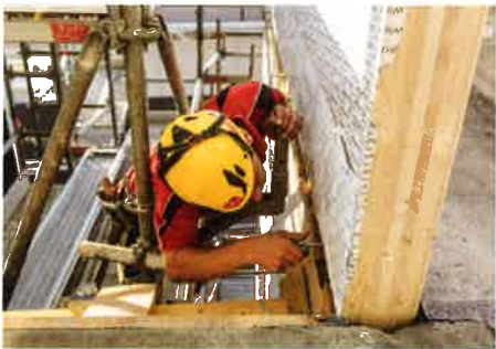
Sequence of placement and installation of the prefabricated wall panels. The bottom right image shows the installation of an interior core free-standing column.
