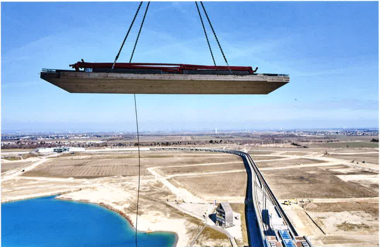
Floor panel with pre-installed mechanical services element
